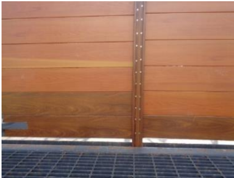
Photo No. 3 Panels Installed to Center Post
