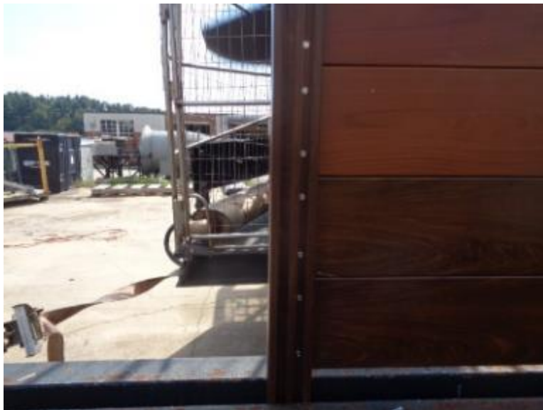
Photo No. 4 Panels Installed to End Post
